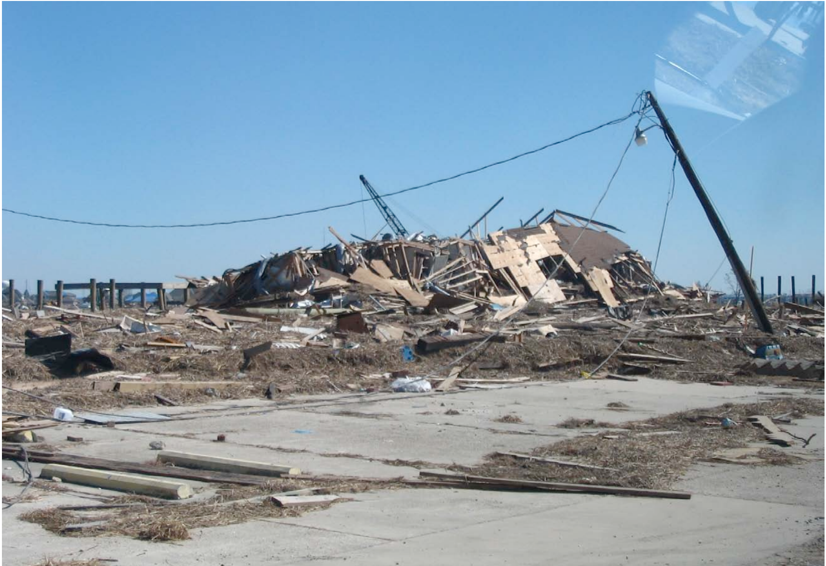
This was a house. No bulldozer involved. Slidell, LA - October 16, 2005
