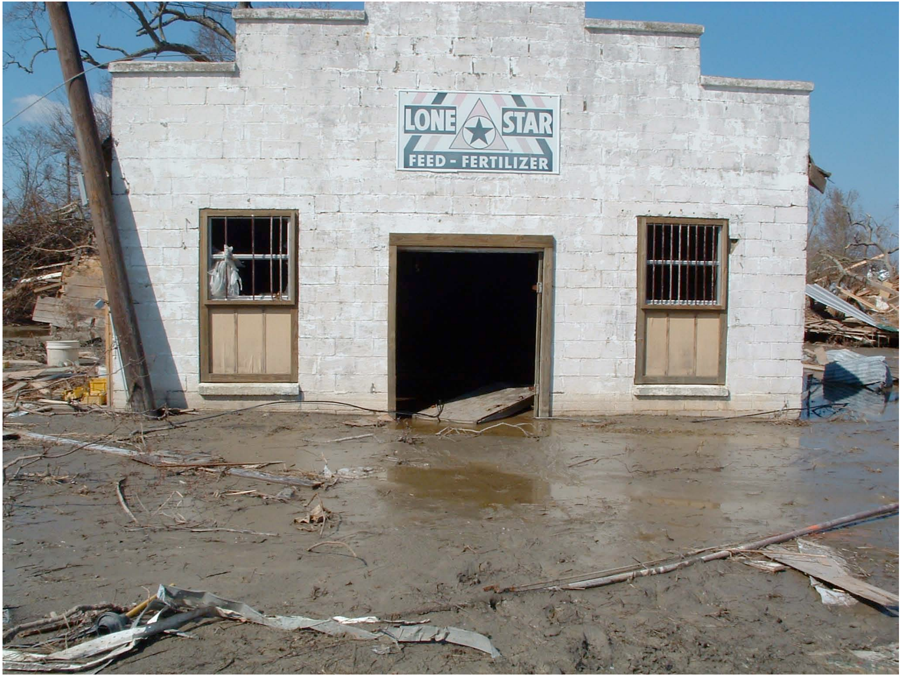
Little bit of mud. Creole, La Highway 1143
