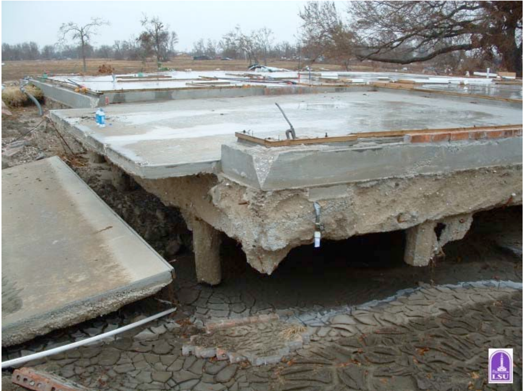
Storm-surge scour revealed foundation
