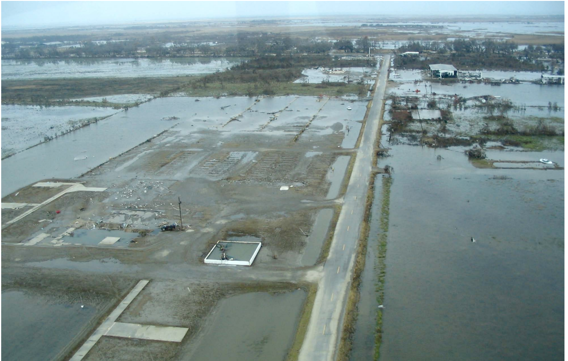
Cameron, La. below highway 82 - September 28, 2005
