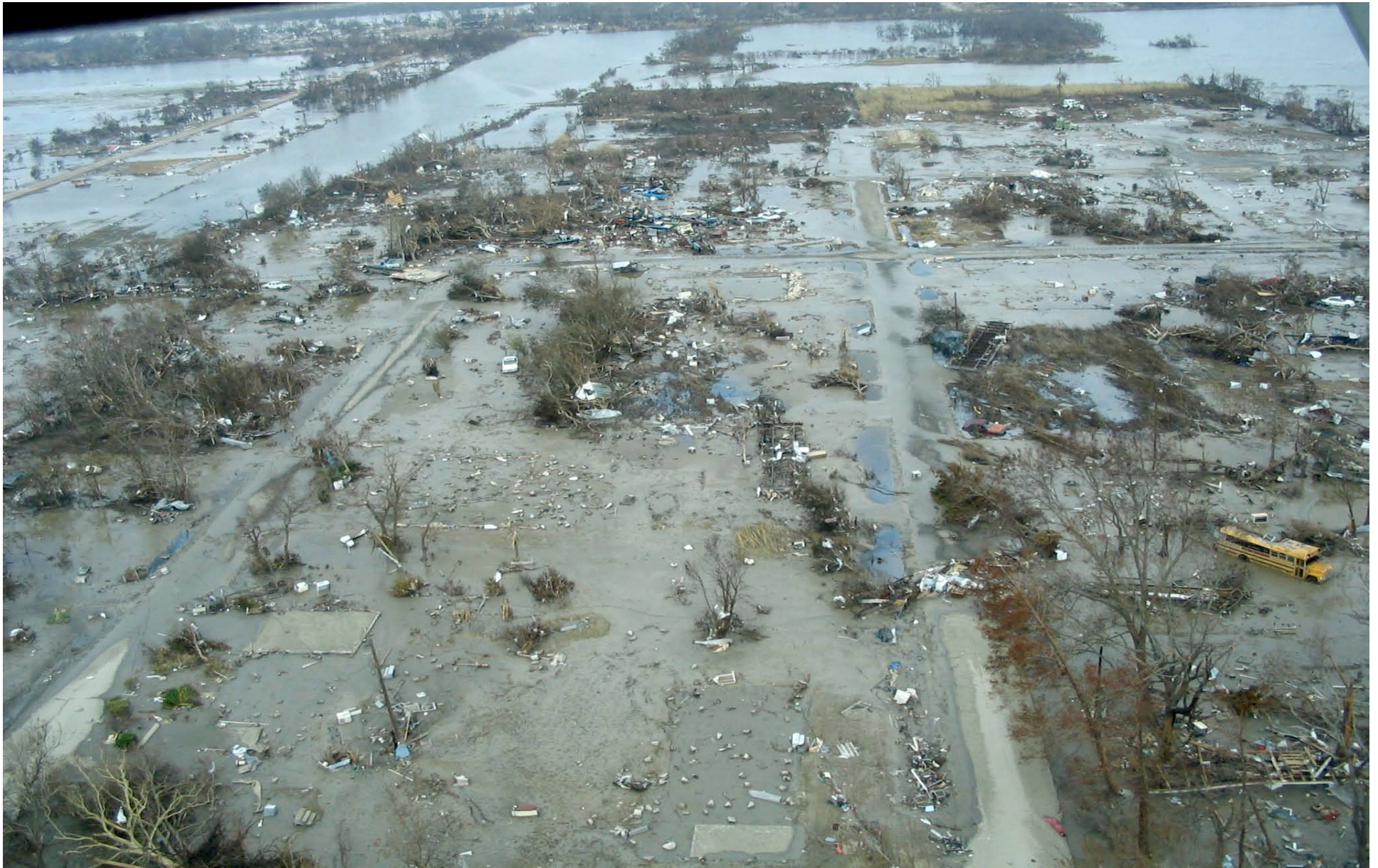
Cameron, La. below highway 82 near 1142 - September 28, 2005
