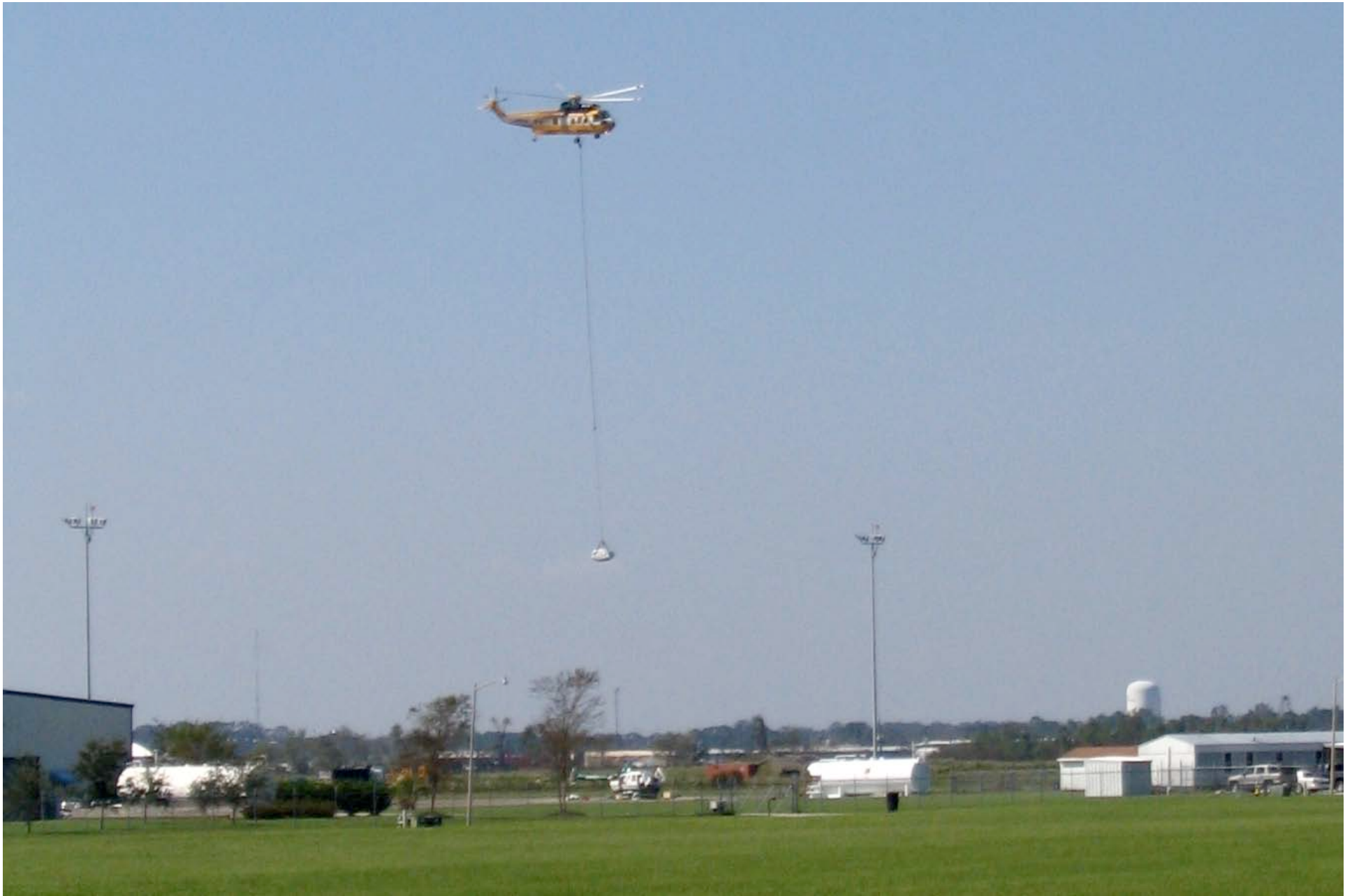
Repairing the Houma levee - September 28, 2005
