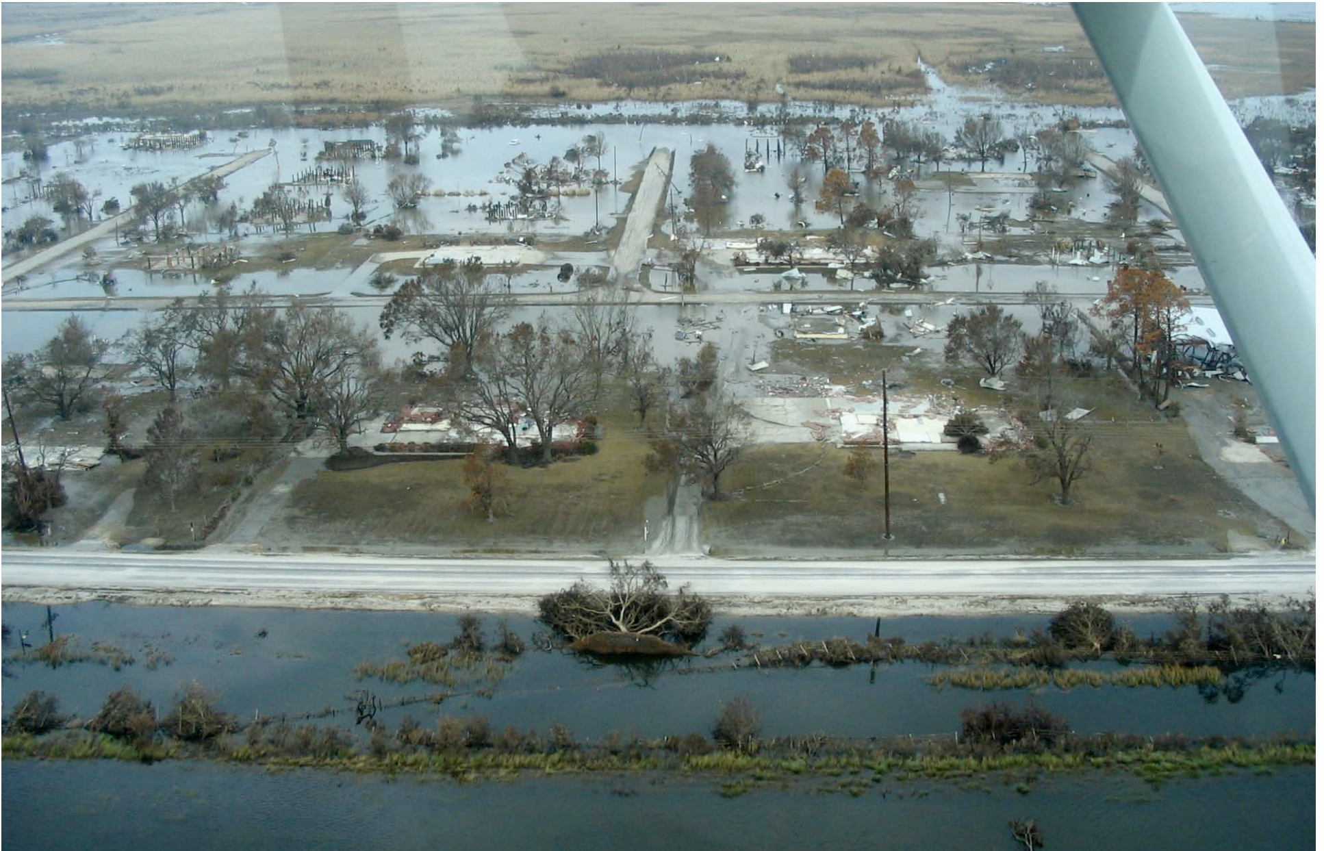
Cameron, La. along highway 82 - September 28, 2005
