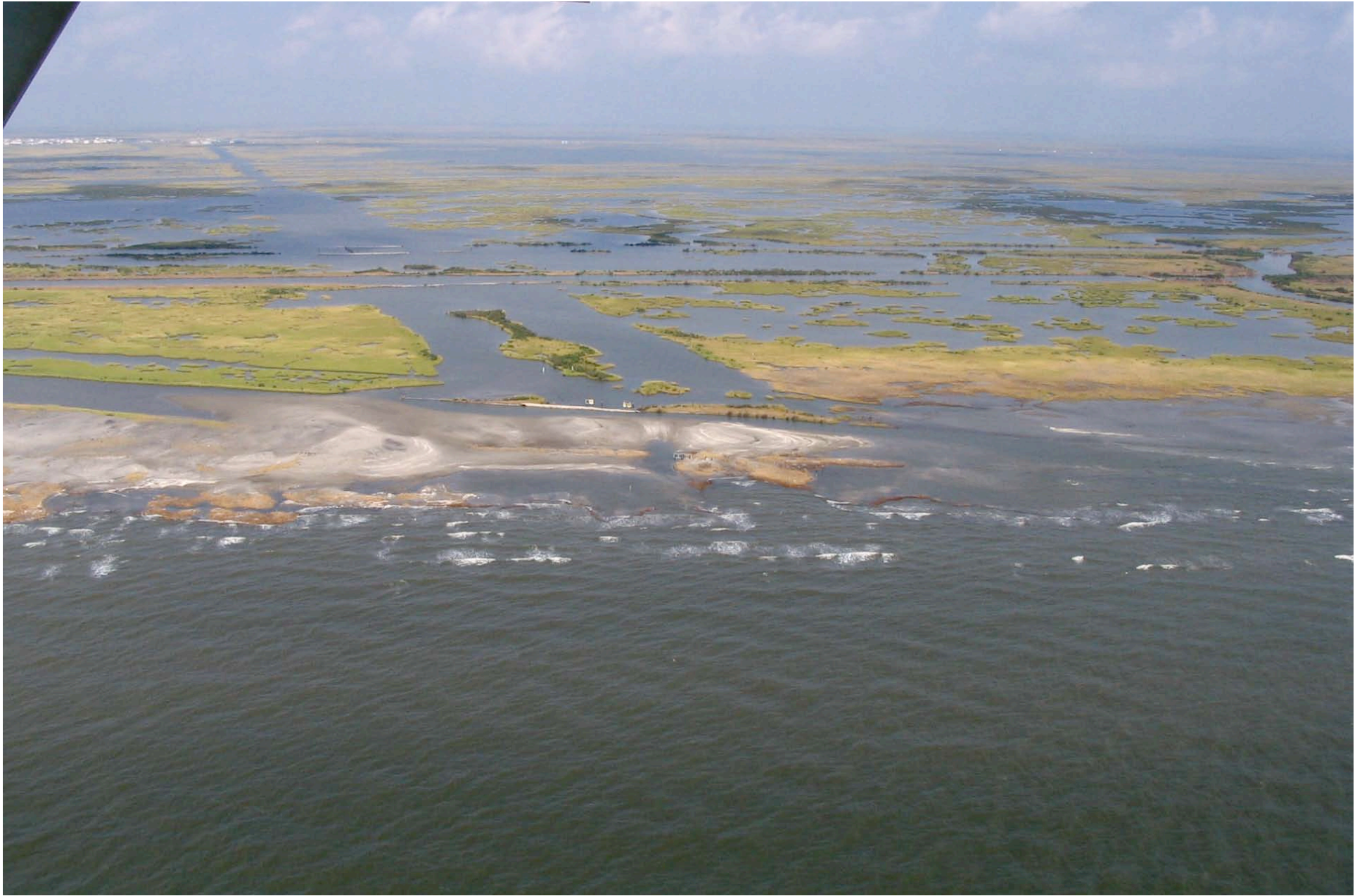
LOOP pipeline; Caminada Headland - September 30, 2005
