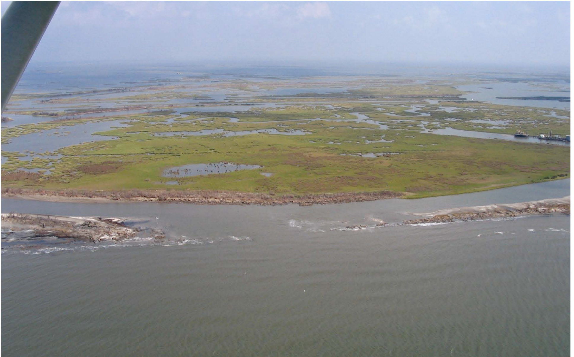
Breach into access canals west of Bay Chaland - September 30, 2005
