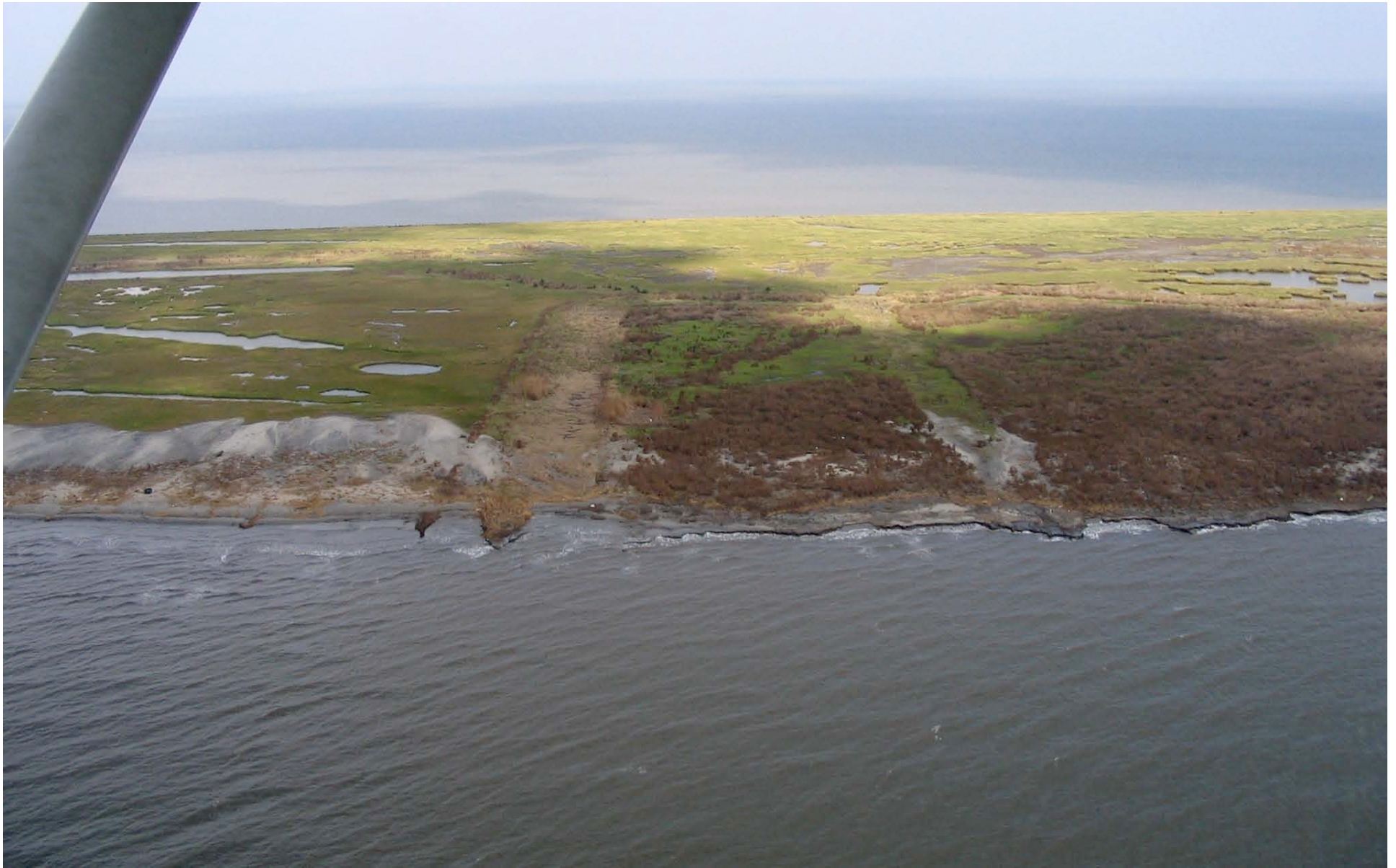
West Grand Terre; natural marshes to the left, restoration area to the right - September 30, 2005
