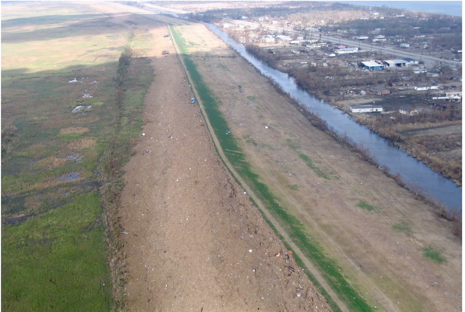
West levee at Venice, LA looking north - September 30, 2005. Notice heavy wrack line against levee
